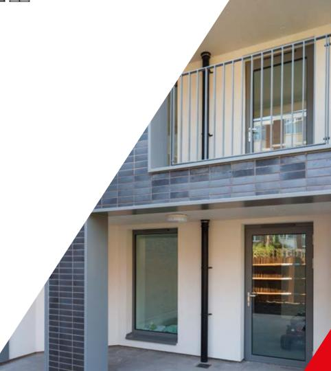
1 U-value in accordance EN 10077-2, single door size 1000mm x 2180mm. 2 U-value in accordance EN 10077-2, double door size 2000mm x 2180mm. U-values based on CEN size door (1000mm x 2180mm) using 1.0 W/m2K double glazing with warm edge Swisspacer V bar. All weather test data taken from BS EN 6375-1 (Part of PAS 23) based upon the highest performing door configuration.
